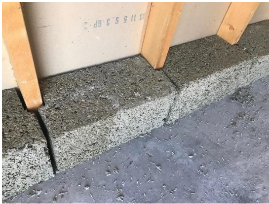
Notched blocks to fit stud framing:
