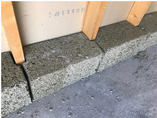
Notched blocks to fit stud framing:
